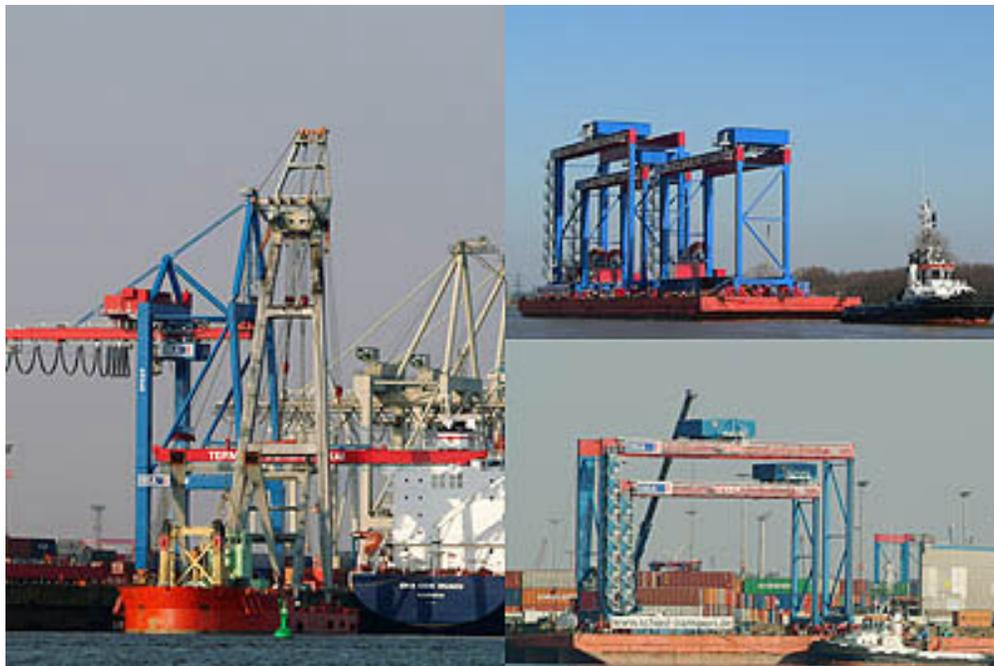
**Crane barge Uglen erects two new gantries at CTB, while more and more Kalmar-built constackers arrive by barge. Photos: Willy Thiel (1), Jan Tiedemann (2)**
